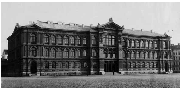
fig.2 Façade of the Ateneum building, 1890 Finnish National Gallery, Archive Collections. The University of Helsinki Department of Art History Donation Collection. Photographer: Daniel Nyblin, Helsinki
